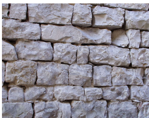
Mur : limousinage (Naves)
